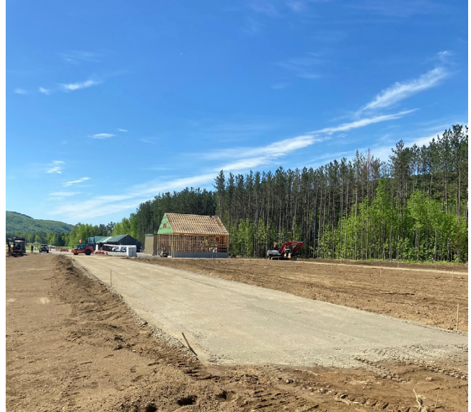
Airport Taxi-Lane Construction - Summer 2022
