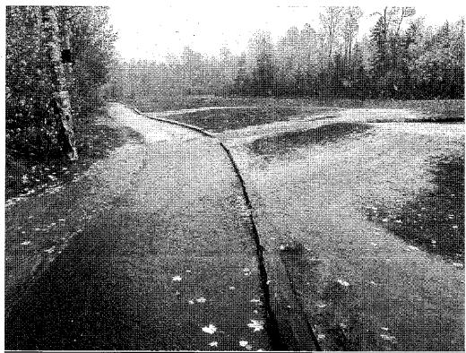
Cross drainage on #2 - outlet needs a good cleaning of sand and leaves to keep drain flowing
