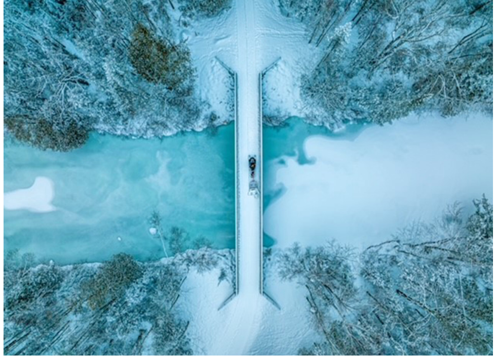
Campbell Field Bridge - Photo credit Samuel Trafton
